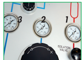
The three pressure gauges indicate:
