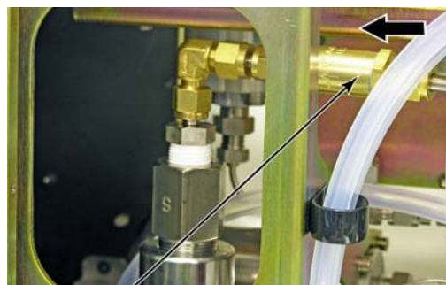
PUMP INLET FILTER (LIQUID)
